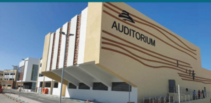
Lycée School - Abu Dhabi, UAE
